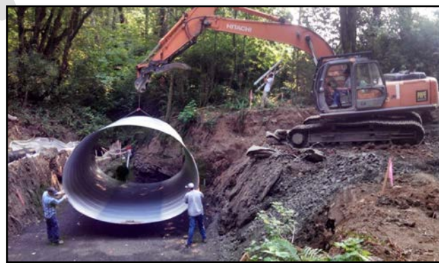
Figure 9. Voluntary culvert replacement to improve fish passage.
