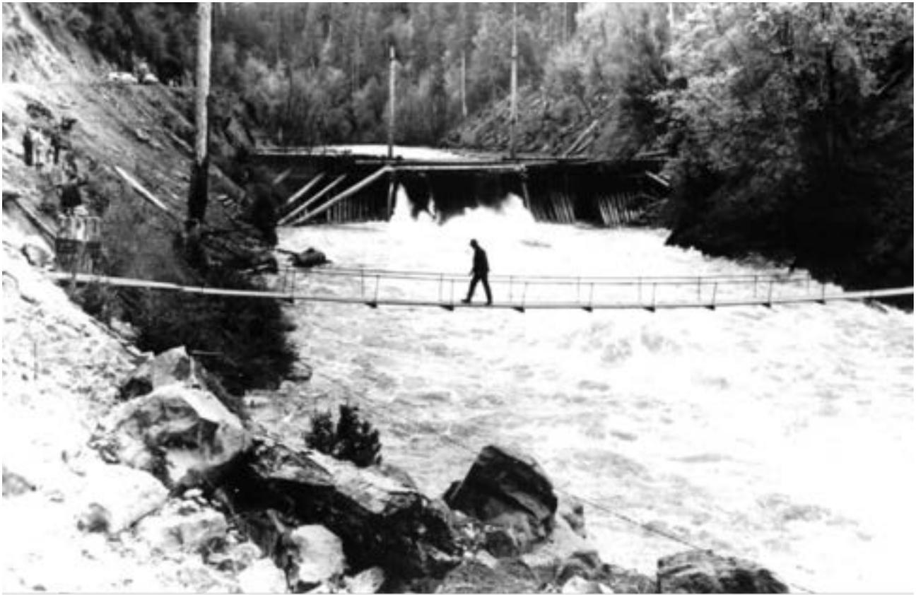
**Figure 3-5.** The largest and last operating splash dam in the Pacific Northwest was the Tioga Dam, located on the South Fork of the Coos River in Coos County, Oregon. Circa 1957. Photo: Bill Wilt.
