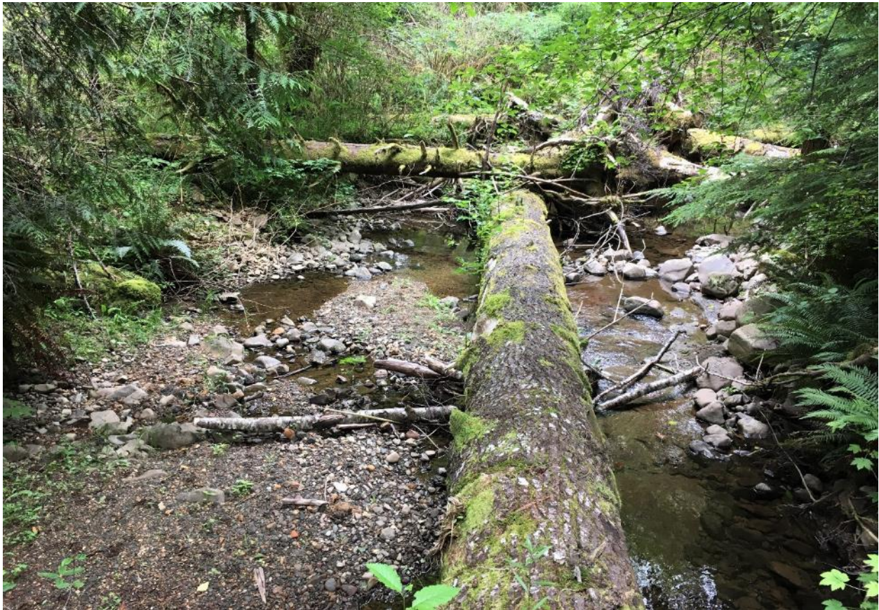
Photo 105 Jack Horner Bedload Accumulation Associated with LWD Structure
