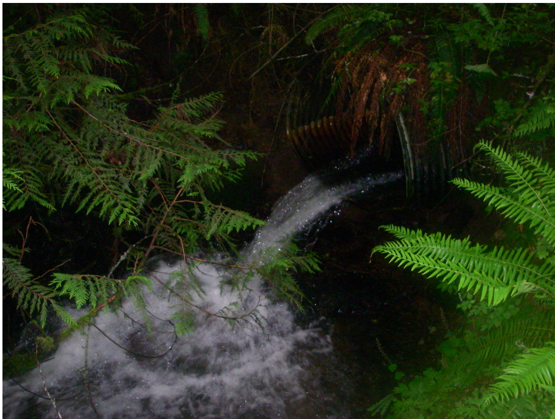
Photo 19. Culvert in Trib A of Selder Cr.
