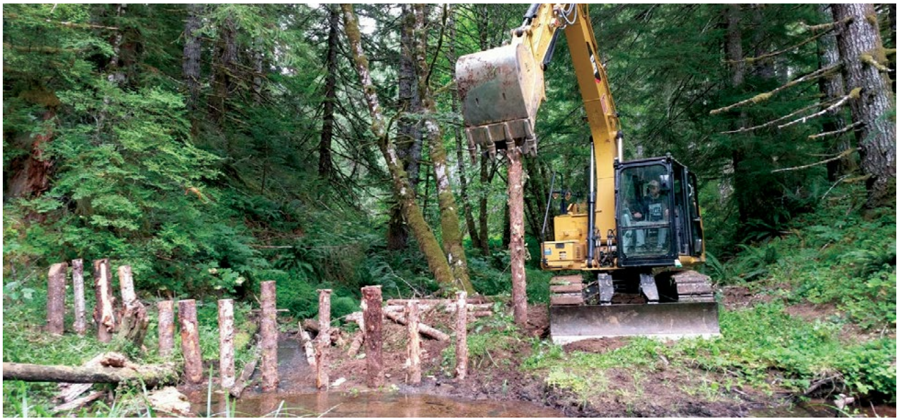
Beaver Dam Analogues are wood structures that can mimic beaver dam construction. Photo: Maggie Peyton
