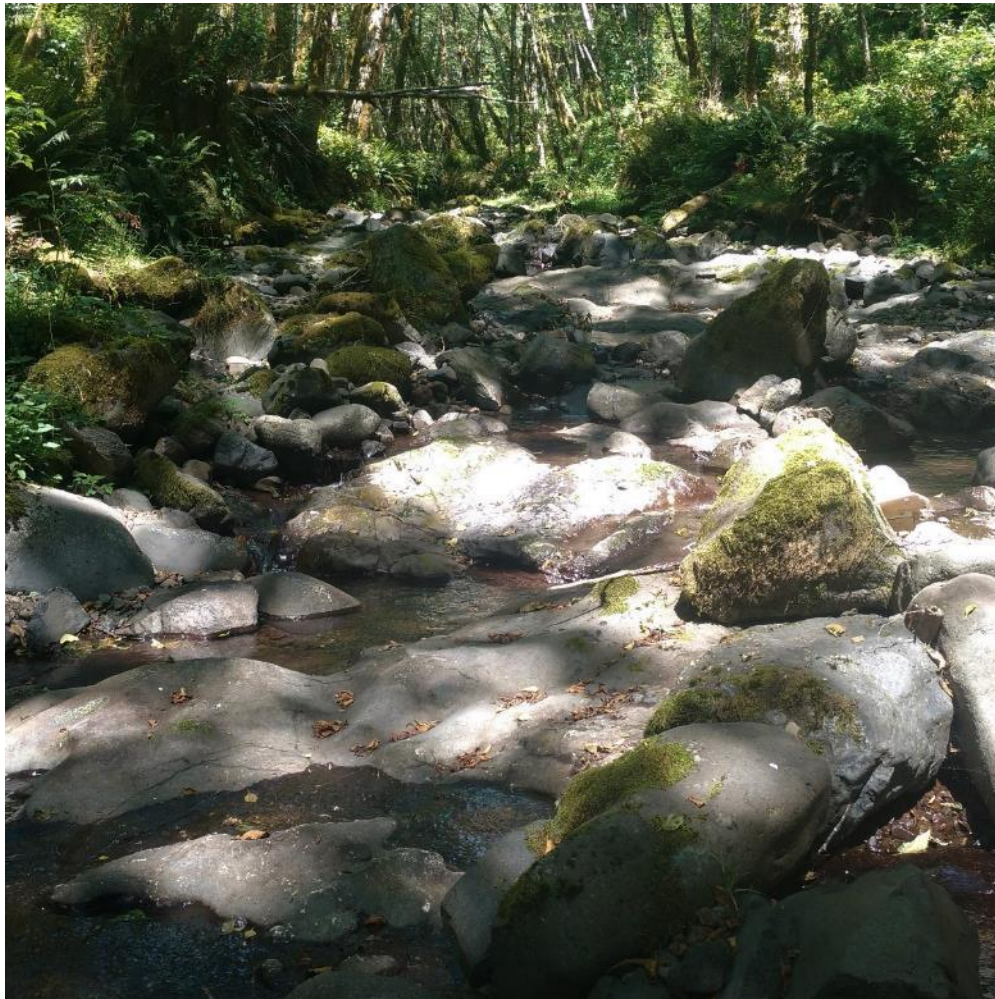
Photo 14 Bastard Creek Scoured Bedrock and Boulders
