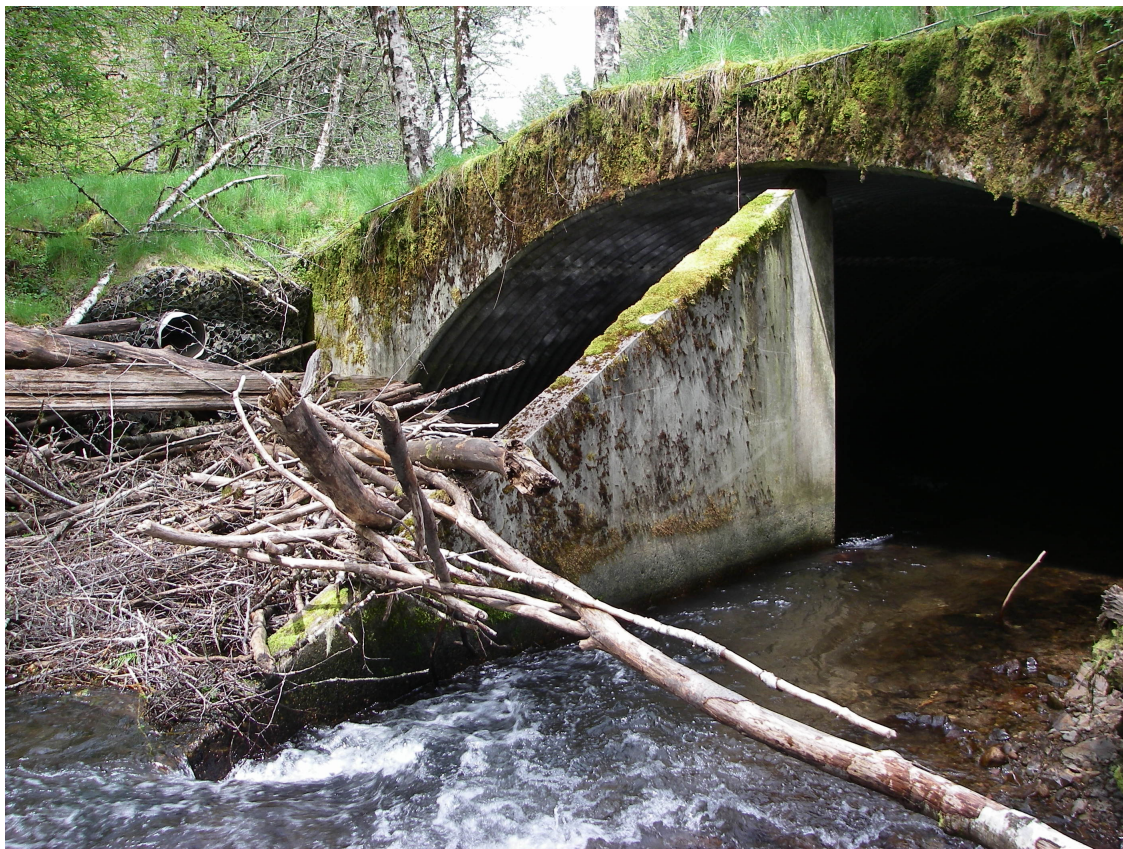
Photo 6. Hwy 26 culvert SF Rock.
