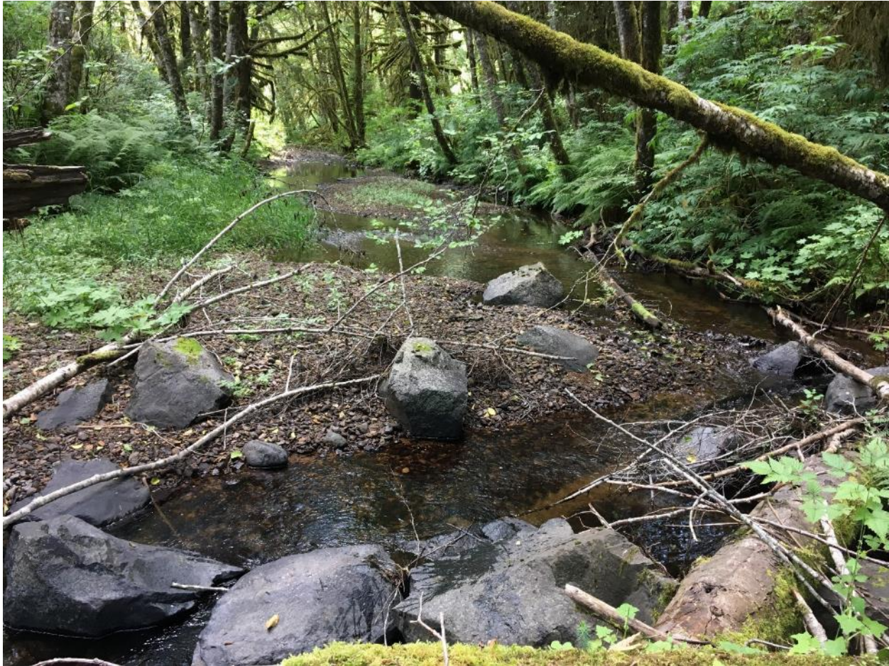
Photo 117 Fall Creek Boulder Weir Impounding Gravel
