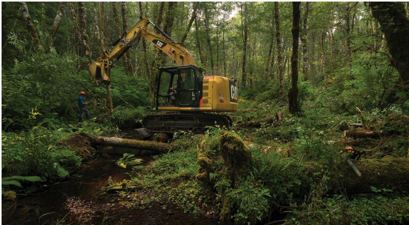
The installation of large wood can boost short-term Coho production and enhance watershed function. Photo: Dave Herasimtschuk
